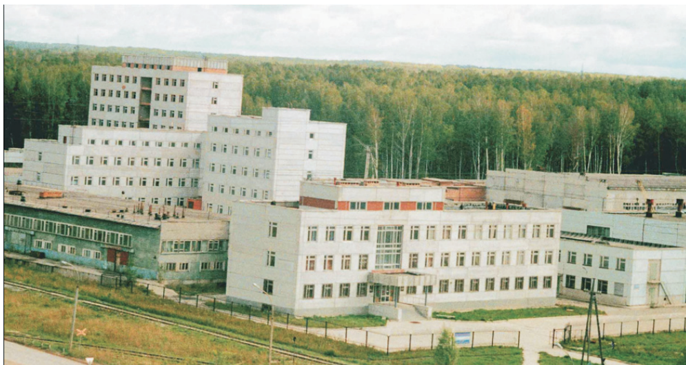
Institute of Solid State Chemistry and Mechanochemistry SB RAS (Novosibirsk). These buildings were built thanks to the efforts of Prof. V. V. Boldyrev, when he was the Director of this Institute
